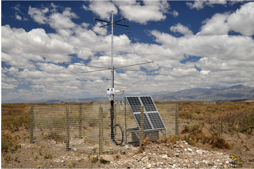
Figure 4.8: AERA station with wired LPDA.
