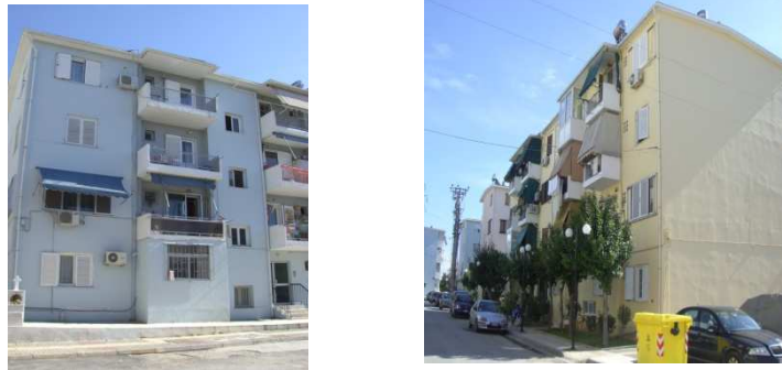
Figure 1 Buildings R7, R8
