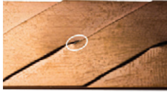
Figure 6.8: Damaged sections of the 10 strand RACC (no epoxy impregnation) after in-field measurements in worst case field orientation.
