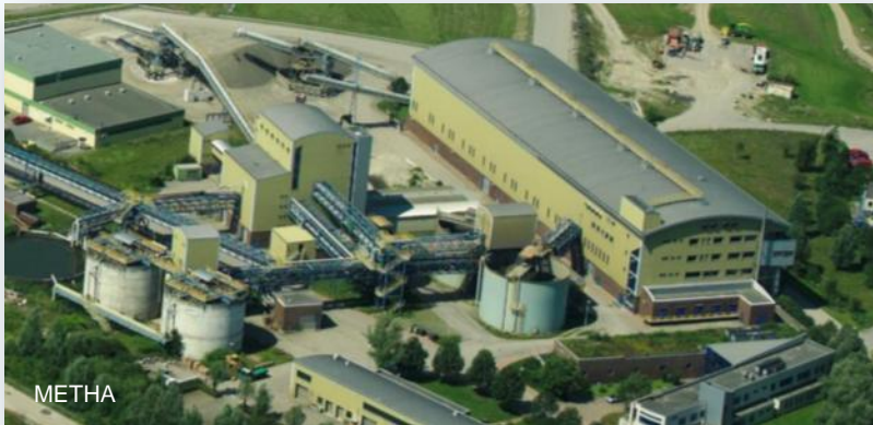
METHA Treatment facility
