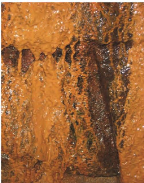
**Figure 2:** Rusty orange to brown *Gallionella ferruginea* dominated biofilms, attached to the fractured bedrock of the Äspö HRL tunnel.
