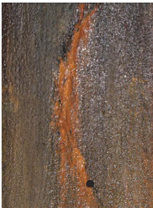
**Figure 1:** Rusty orange to brown *Gallionella ferruginea* dominated biofilms, attached to the fractured bedrock of the Äspö HRL tunnel.
