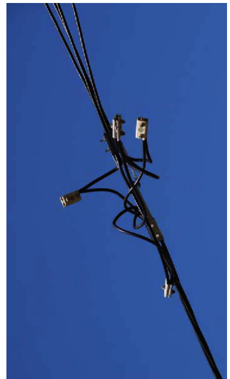
Abb. 13: Provisorisch reparierte Stromleitungen Quelle: Final Report, Damage Assessment and Needs Identification in the Gaza Strip, 3/2009
