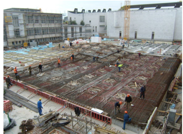
Abb. 18 Baustelle, November 2011 © Bollinger + Grohmann
