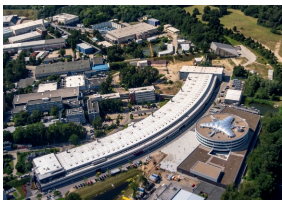
Figure 1 Aerial view of the almost 300 m long PETRA III experimental hall "Max von Laue" 2012.
