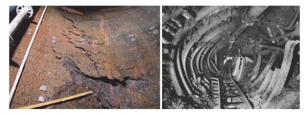
Fig. 4: Breakouts in tunnel walls can lead to loss of lives or require expensive safety measures. Left: fractures in a shaft wall in the Äspö rock mechanics laboratory in Sweden. Right: tunnel wall deformation in the Lignite Mine near Peissenberg, Germany.
