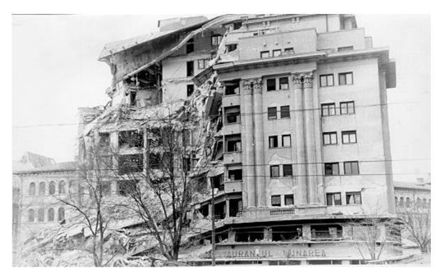
Partially collapsed building in Bucharest after the March 4, 1977 earthquake (Foto courtesy D. Lungu)
