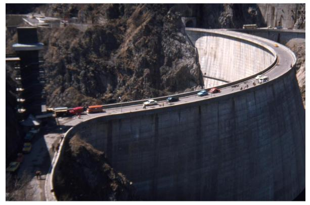
Fig. 13: The double curvature arch dam Vidraru-Arges. The station ARS was installed in the area of the eastern abutment (left side) of the dam. The red VW-Bus of the GPI is parked at the left side of the dam.
