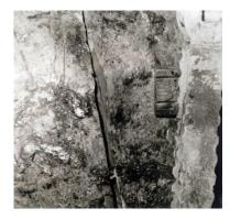
Fig. 6: Hydraulic Fractures in a coal mine in Saarland region. The hydraulically produced fractures have been reached by the mine trajectory (RAG-Archiv Saar).
