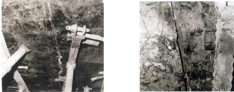
Fig. 6: Hydraulic Fractures in a coal mine in Saarland region. The hydraulically produced fractures have been reached by the mine trajectory (RAG-Archiv Saar).
