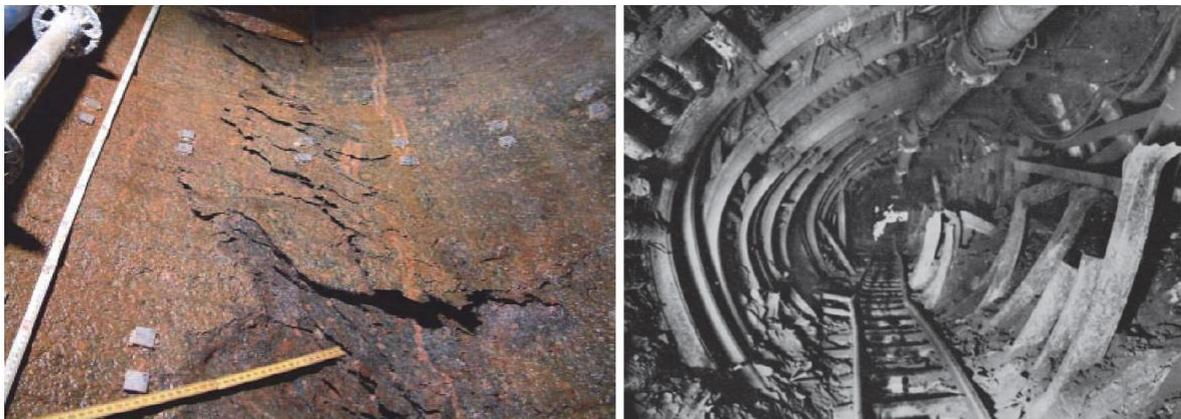
Fig. 4: Breakouts in tunnel walls can lead to loss of lives or require expensive safety measures. Left: fractures in a shaft wall in the Äspö rock mechanics laboratory in Sweden. Right: tunnel wall deformation in the Lignite Mine near Peissenberg, Germany.
