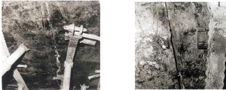
Fig. 6: Hydraulic Fractures in a coal mine in Saarland region. The hydraulically produced fractures have been reached by the mine trajectory (RAG-Archiv Saar).
