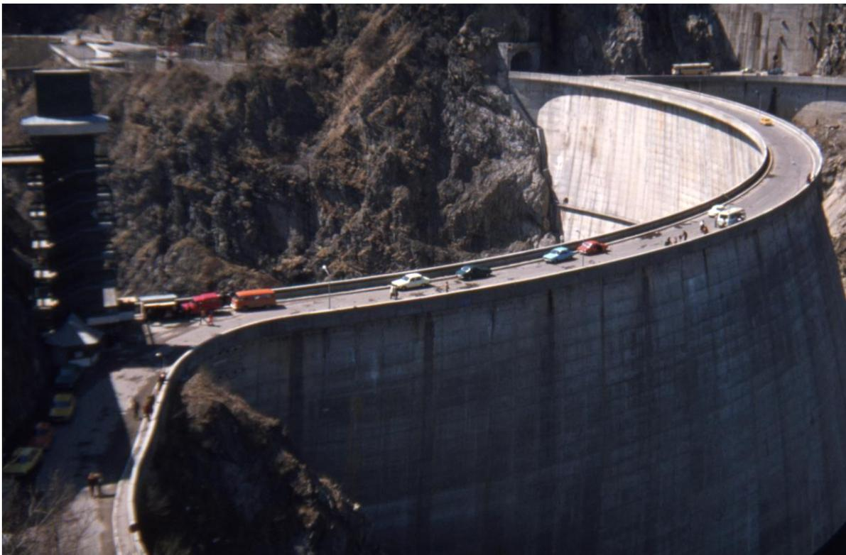
**Fig. 13:** The double curvature arch dam Vidraru-Argeș. The station ARS was installed in the area of the eastern abutment (left side) of the dam. The red VW-Bus of the GPI is parked at the left side of the dam.
