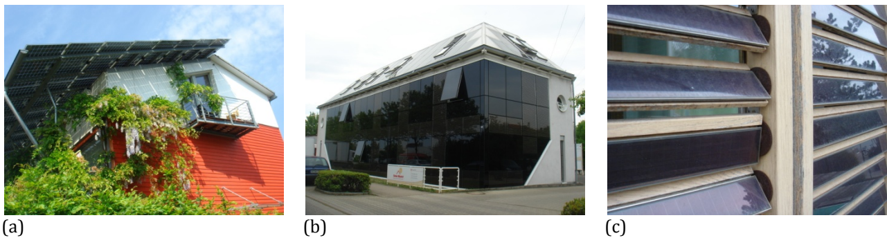
Figure 2.3: Examples of PV application for roofs (a), facades (b) and sunshades (c).
