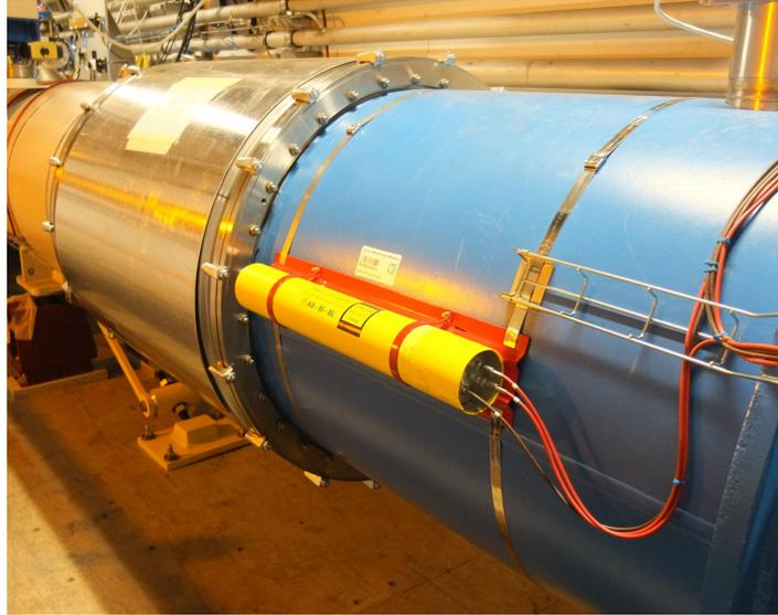
Figure 2.3.: A beam loss monitor tube installed at a dipole magnet.
