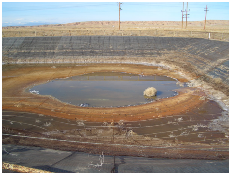
(d) Dried out collection/evaporation reservoir with plastic foil
