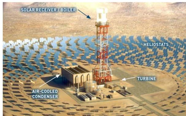
Figure 5: The Ivanpah solar plant in California is the world's biggest. It has a capacity of almost 400 megawatts (MW) and more than 347,000 mirrors focus on three tall towers, which contain water (<http://www.theatlantic.com/infocus/2014/03/the-ivanpah-solar-electric-generating-system/100692/>)(1)
