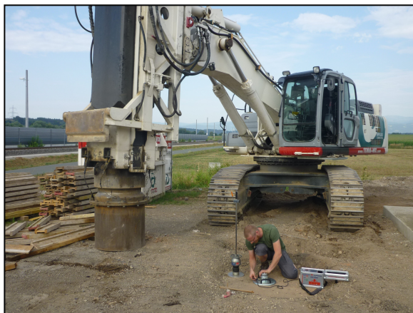
Fig. 6. Rapid Impact Compactor
