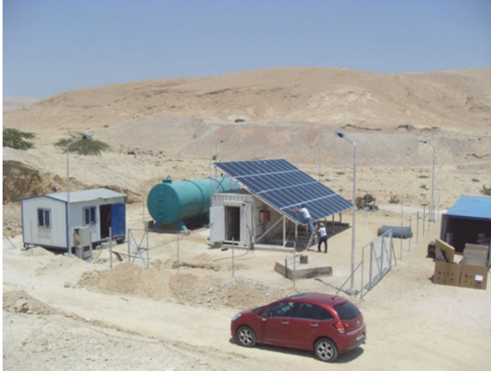
Figure 109: Installation of the solar power plant in Karameh (photo: SPA).
