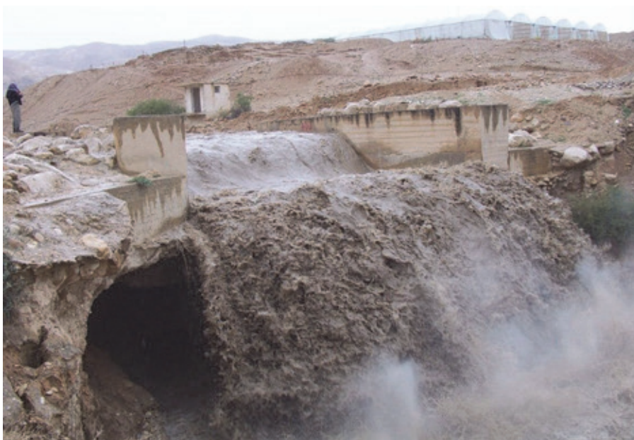
Figure 4: Flash flood event in Wadi Qilt on March 1, 2012 (Picture: courtesy of Palestinian Water Authority). The runoff at time the picture was taken was about 23 \text{ m}^3 \text{ s}^{-1} .
