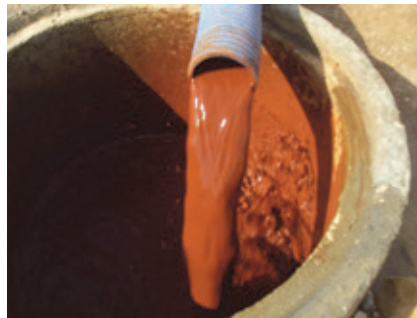
Figure 110: Well water after stop and restart of the well pump (photo: SPA).
