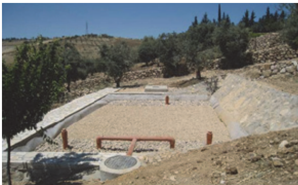
Figure 49: Sequencing batch reactors of Mr Al Hadidi.
