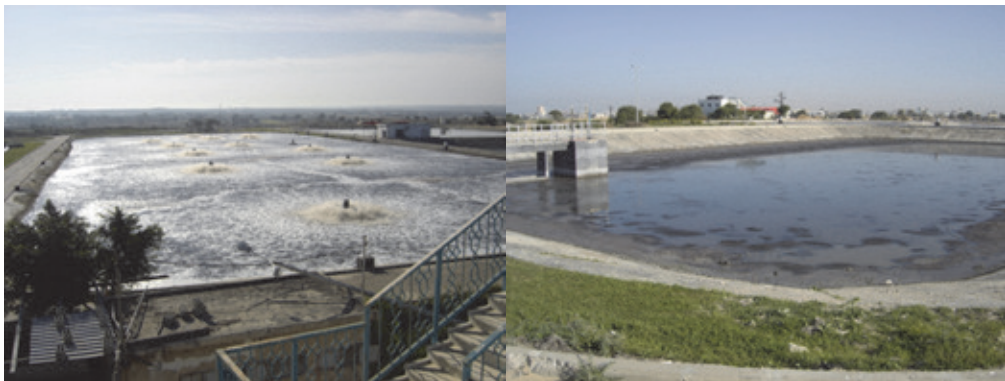
Figure 194: Gaza wastewater treatment plant: Left – aerobic pond; right – sludge holding pond/drying lagoon.
