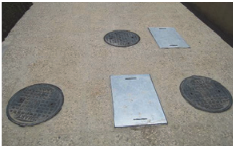
Figure 45: Modified septic tank of MR SHEHABI
