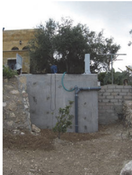
Figure 48: Sequencing Batch reactors of Mr Al Awamleh
