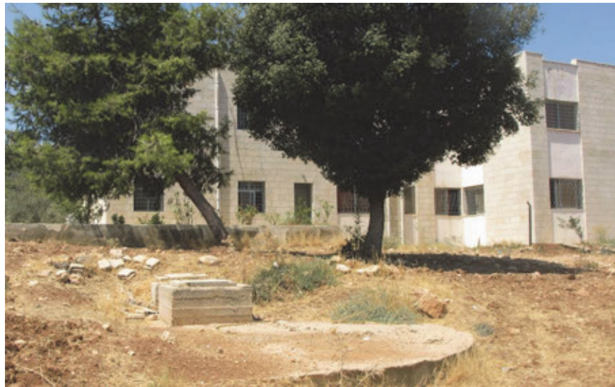
Figure 52: The treatment Wetland at Princess Rahmeh College, Zay
