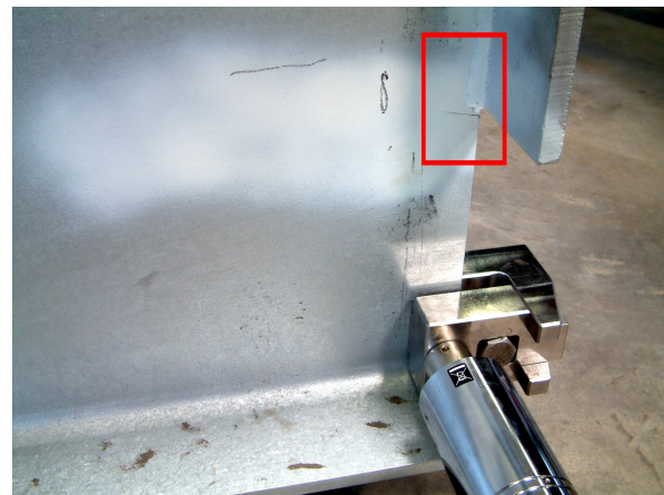
(b) Clamped transducer and marked crack location
