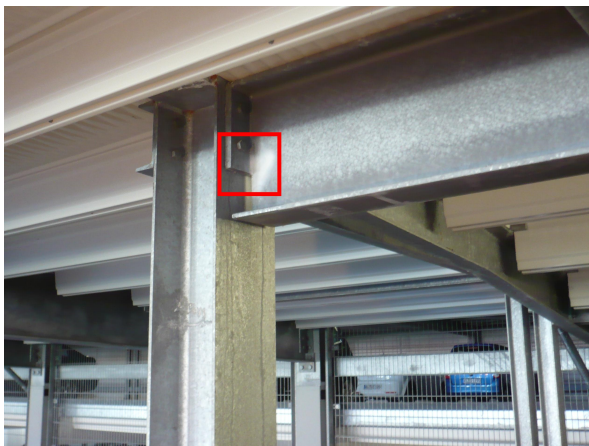
Zinc-coated steel girder with attached head plate in a multi-storey car park
