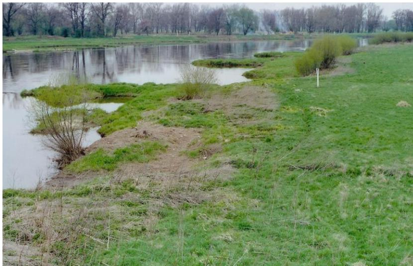
Figure 2: Groyne basins at Ścinawa (Steinau) in the middle Odra river reach are filled partially with deposits up to 2 m thick.
