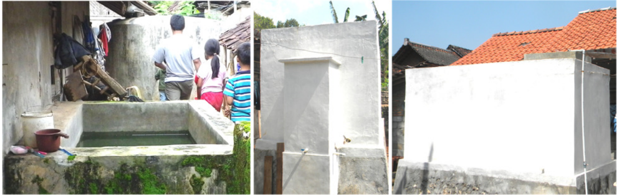
Figure 6: Left: traditional open tank. Middle and Right: optimized covered tank with gravel filter.
