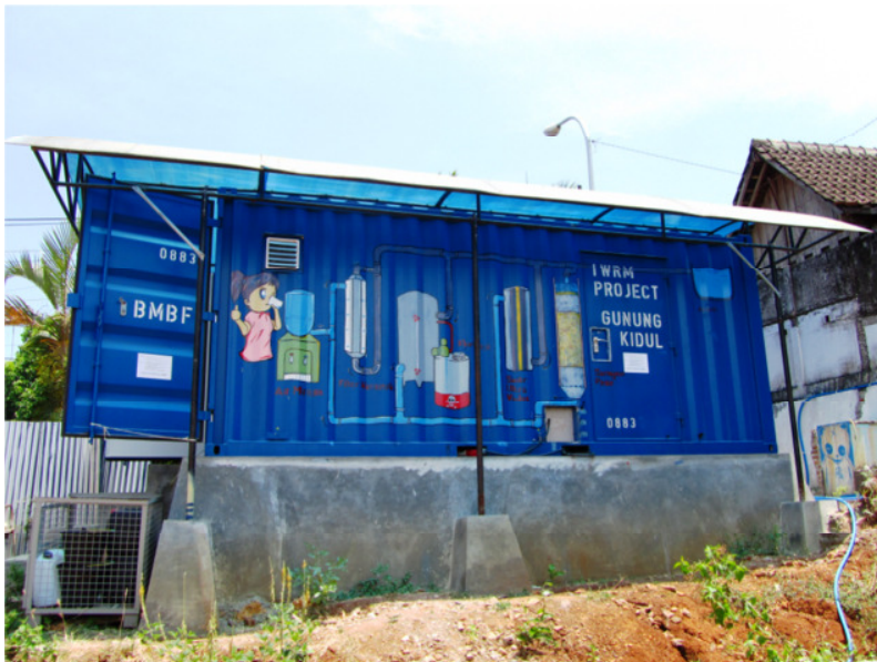
Figure 5: Field laboratory installed at Hospital Wonosari.
