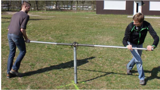
Figure 8. Turning an earth screw into the ground
