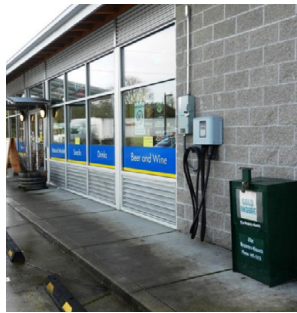
Figure 9.10.: Bad example of a spatial configuration where the charging cable crosses the sidewalk [673]
