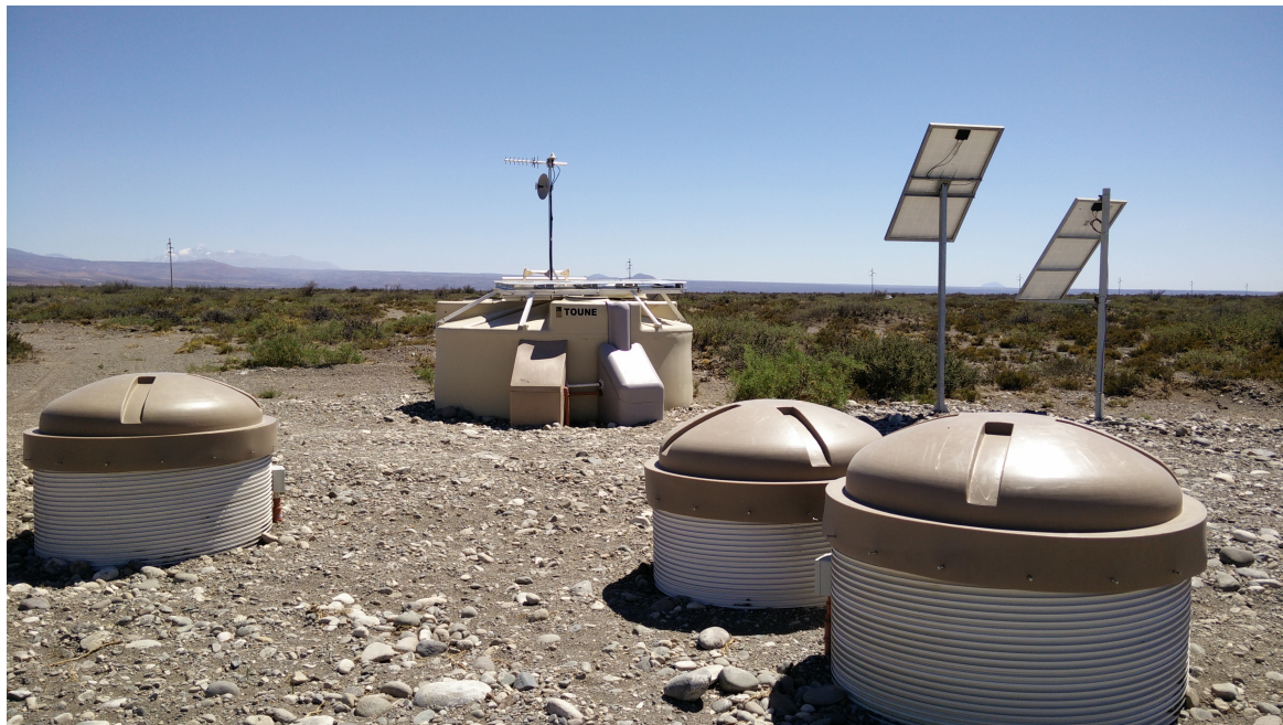
Figure 1.11: The SD-750 station Kathy Turner (Id 1764) with an ASCII 13 2 m 2 prototype mounted on top (see Section 1.2.7). Also visible are additional solar panels and batteries to cope with the increased power consumption. Three AMIGA 14 access tubes are visible in the forefront (personal photograph, November 2014).
