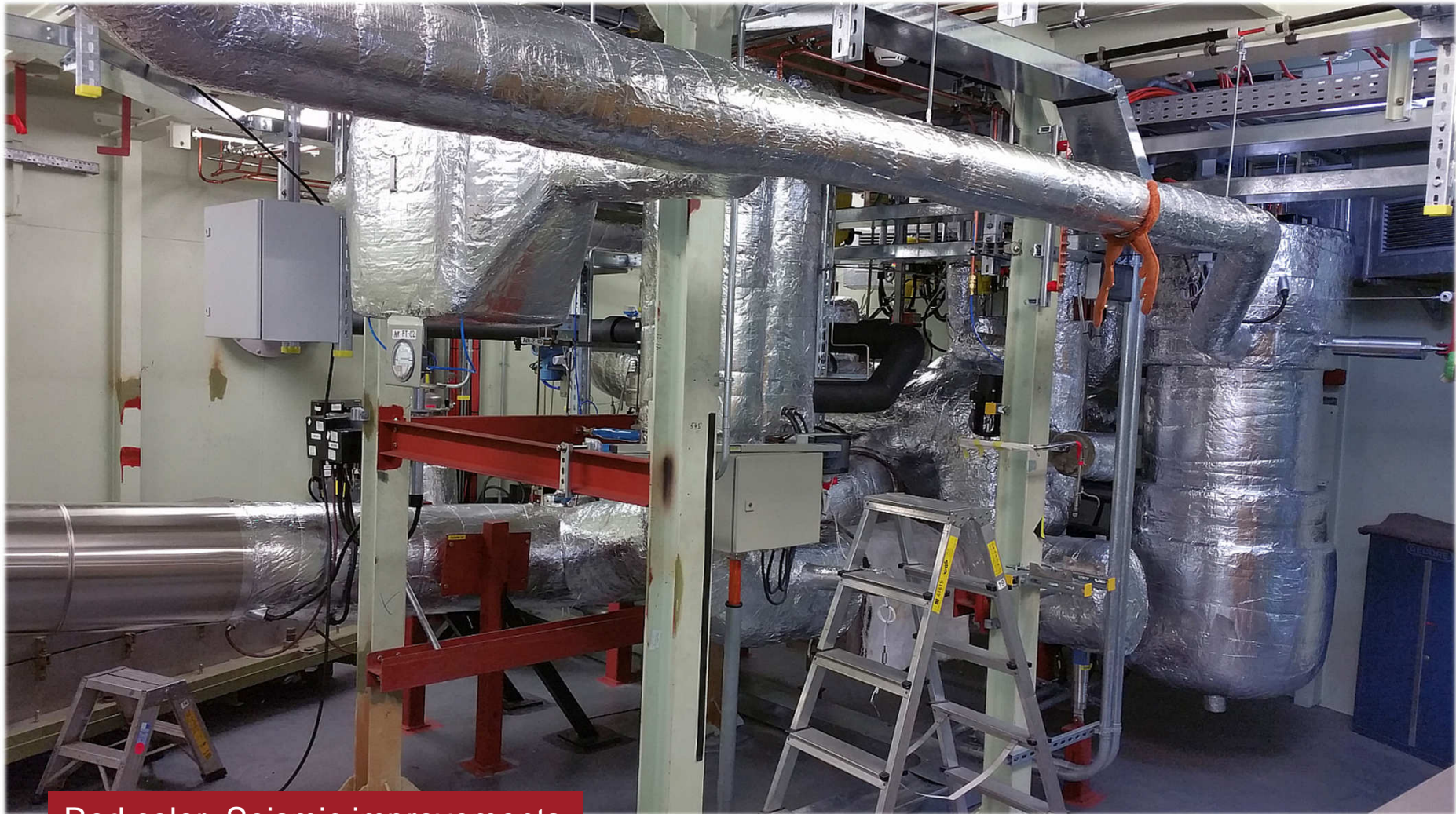
Red color: Seismic improvements
