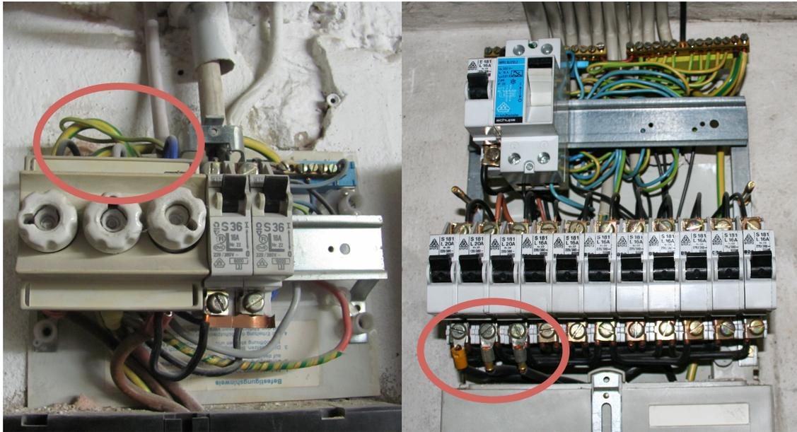
Figure 5.2: Two examples of fuseboxes showing the clearance to the main wires marked with red circles. The left example has enough room for the current transformers while the right one is too restricted.
