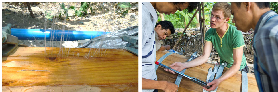
Fig. 4 Illustration of the working steps for the construction of a wood stave pipeline
