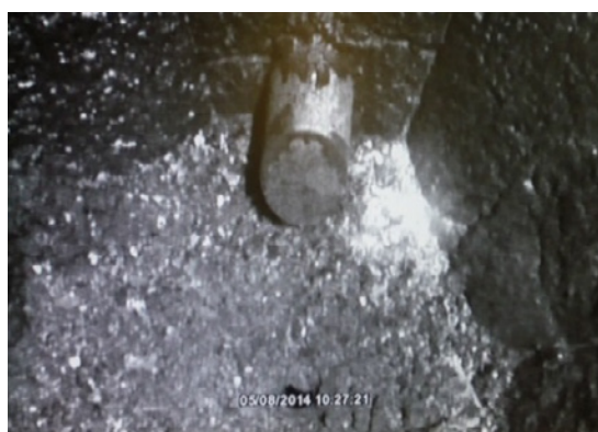
Fig. 10: View of the melter's interior after emptying showing the lower part of the melt tank with the auxiliary electrodes
