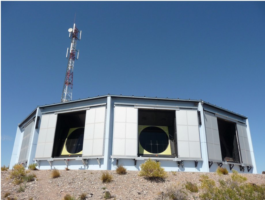
FIG. 2.11 The telescopes at the Los Leones site overlooking the atmosphere above the surface array from atop a small elevation. The telescopes are of course only operated on clear dark nights, but here the shutters were opened for the special occasion of taking this photograph. The communications tower is visible in the background. Photo courtesy of Radomír Šmída.
