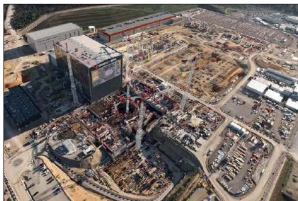
Fig. 1 The ITER site under construction in October 2016 (Photo ITER Organisation/EJF Riche)
