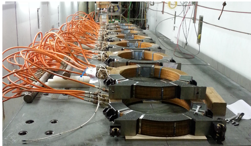
Figure 19: Picture of the staggered coils to produce a strong and uniform magnetic field in the vertical direction to the beam line.
