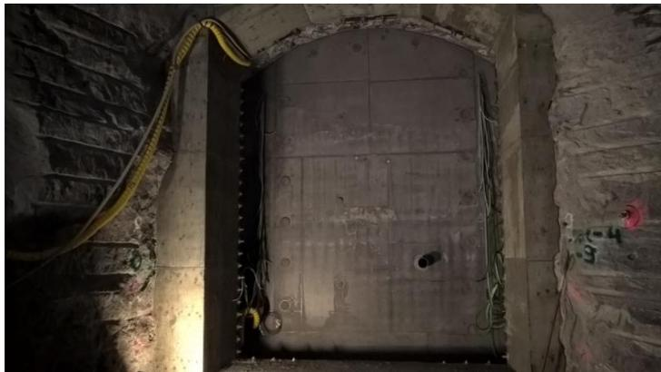
*Figure 1: Deposition tunnel end plug where Posiva's ternary mix design was successfully utilized.*
