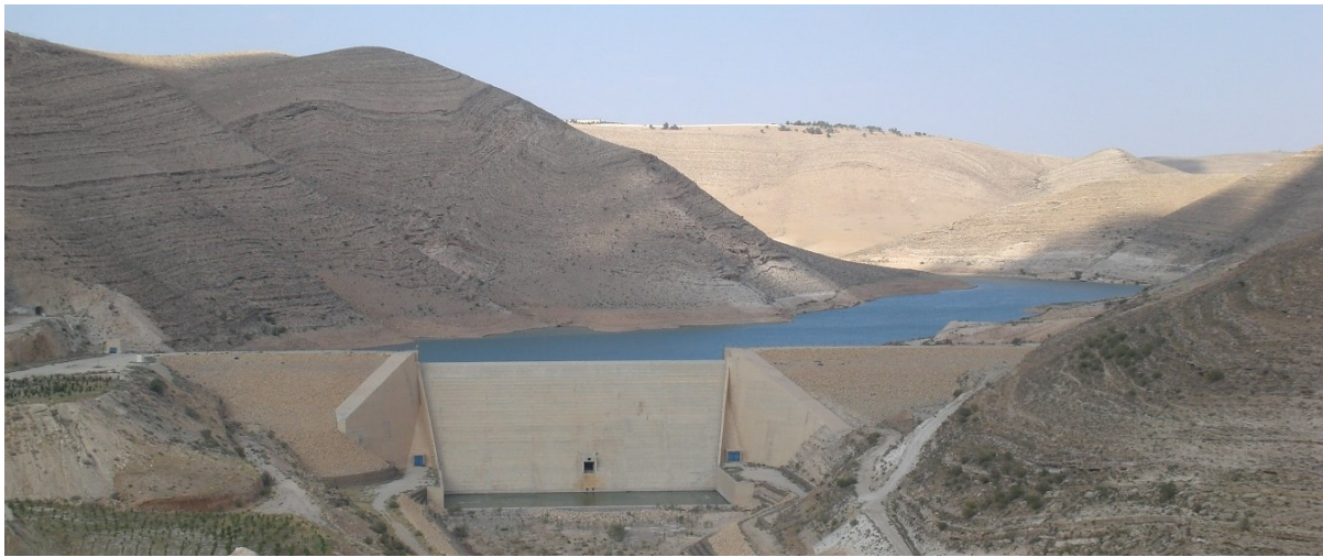
Fig. 1.3 View on the Wala dam, Jordan (Photo: Xanke 2012)
