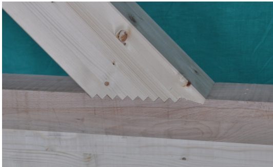
Figure E9-4 Multiple step joint. (Blass and Enders-Comberg, 2012)
