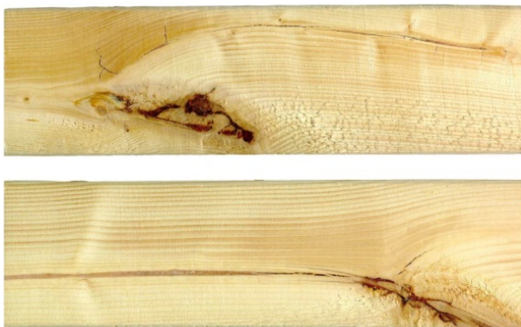
Figure B3-15 Two examples of treetop breakage.
