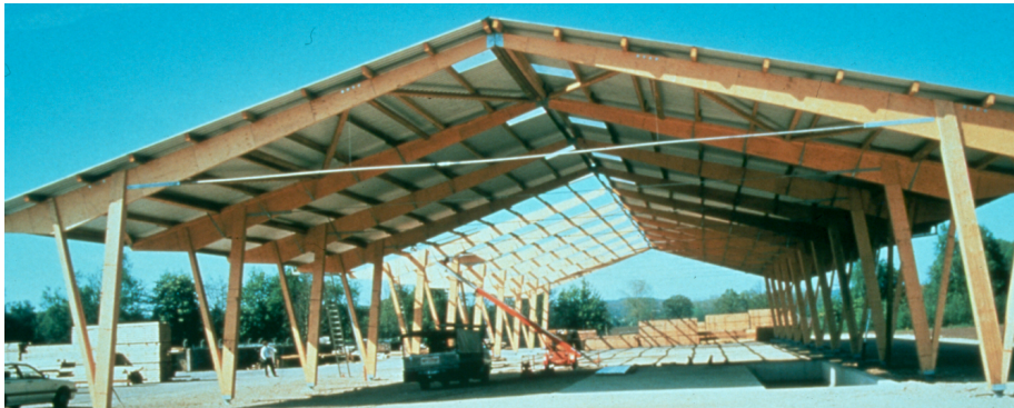
Figure E14-4 Frame corner in a portal frame structure. Division of the corner moment in a tensile and a compressive force. (photo: Finnforest)
