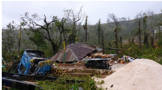
Fig. 1: Devastation in Haiti after Matthew has made landfall. Image source: Engineers Without Borders.
