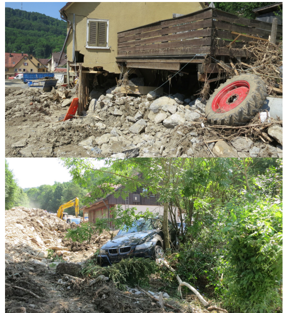
Fig. 2: Structural damage in Braunsbach after the 29 May 2016 flash flood (Image credit: James. E. Daniell).
