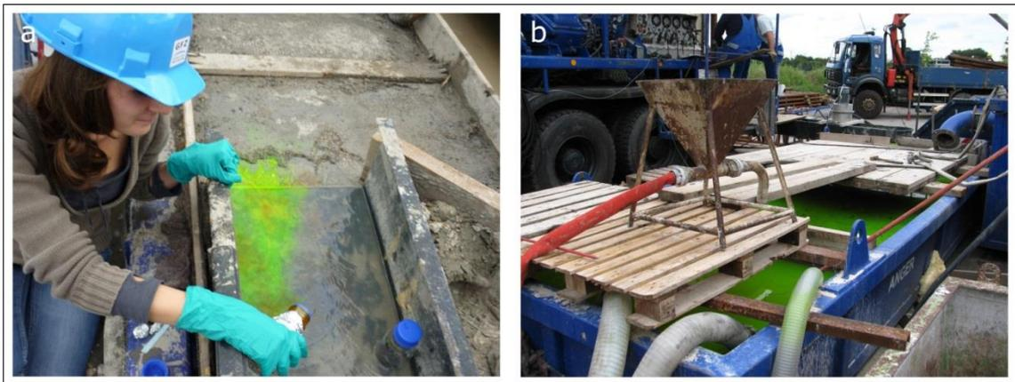
**Fig.8:** Use of fluorescein during the coring of the shallow observation well P300. a: Fluorescein addition into the drill mud tank. b: Green colored drill mud by the incorporation of fluorescein.
