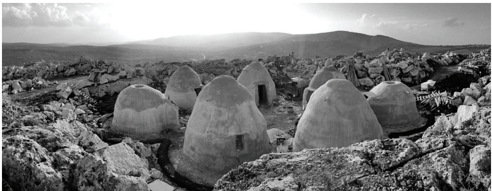
Fig. 1: Sandbag dome shelters in Rif Sarmada, north of Syria; photo courtesy of: Qibaa.
