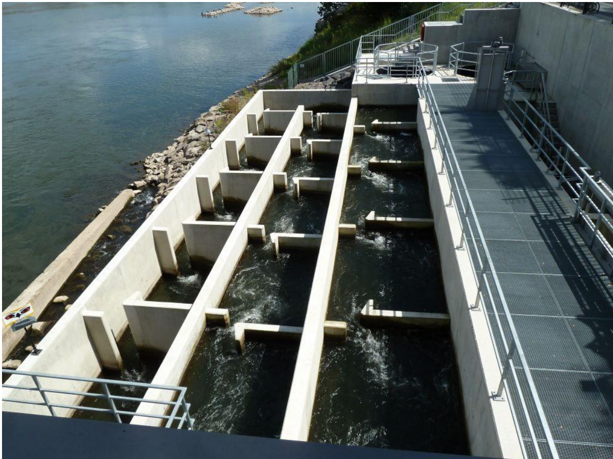
Figure 1.1 View of the vertical-slot fish pass in Koblenz, Germany (Image: BAW)
