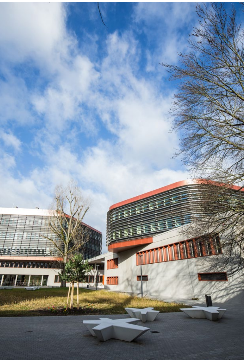
The new Material Research Center on KIT Campus South studies materials for future power supplies.
