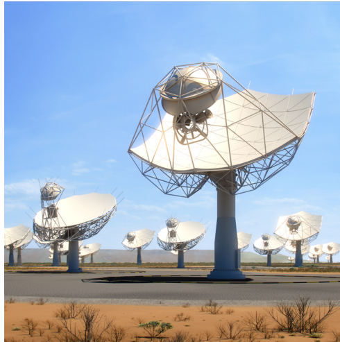
Figure 62: SKA dishes in South Africa (artists rendition, SKA organization). The 15m wide dish telescopes will provide highest-resolution imaging capabilities.
