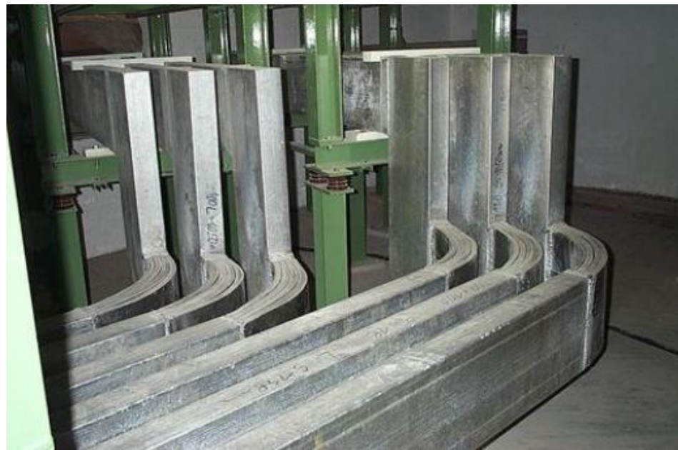
high current bus bar (e.g. for aluminium smelters)
