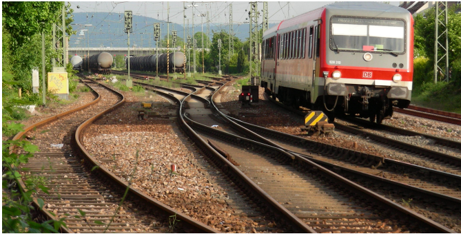
Figure 2.7: Exemplary railway scenario with varying materials. The sleepers of the track on the left side are wooden, whereas those on the center tracks are made of concrete. In addition, ballast and mostly rusted rails can be found, while at most small cross slopes occur (photo by courtesy of Martin Lauer).
