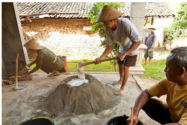
**Fig. 2** Mixing of the mortar in-situ
