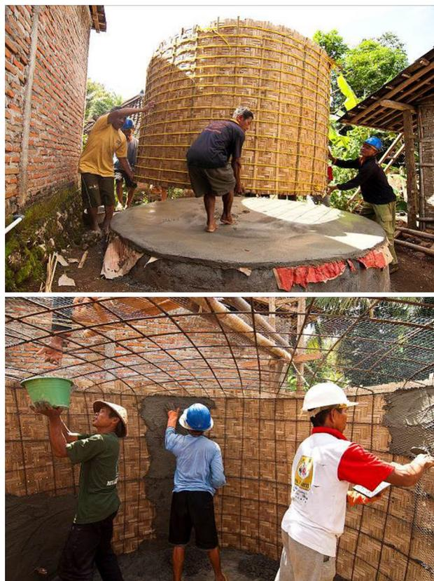
**Fig. 3** Transport of the prefabricated reinforcement cage to the cistern foundation which has been treated with a screed on a decoupling layer of old cement bags before (top) and application of the inner mortar layer (bottom)
