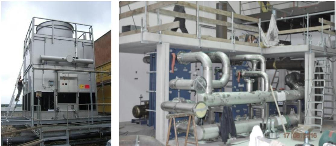
Fig. 1.6.4. 5 MW cooling tower (left) and cooling pipes in FULGOR hall (right).
