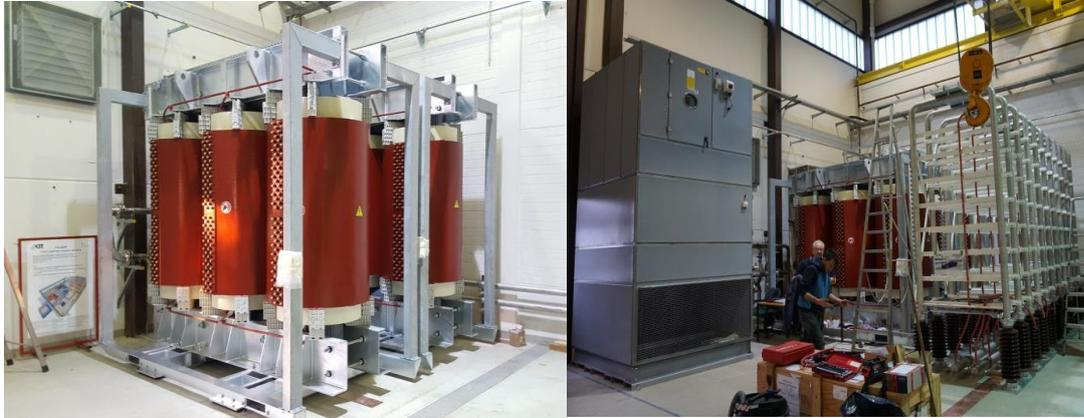
**Fig. 1.6.2:** Left: Two 6.5 MVA transformer installed at FULGOR hall. Right: Ventilation cabin and rack for electronic modules.
