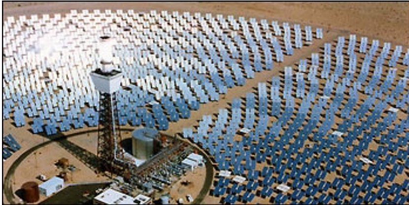
Figure 3.1: Experimental solar power plant Solar Two in the Mojave Desert in California, USA (source: National Renewable Energy Laboratory, USA)
