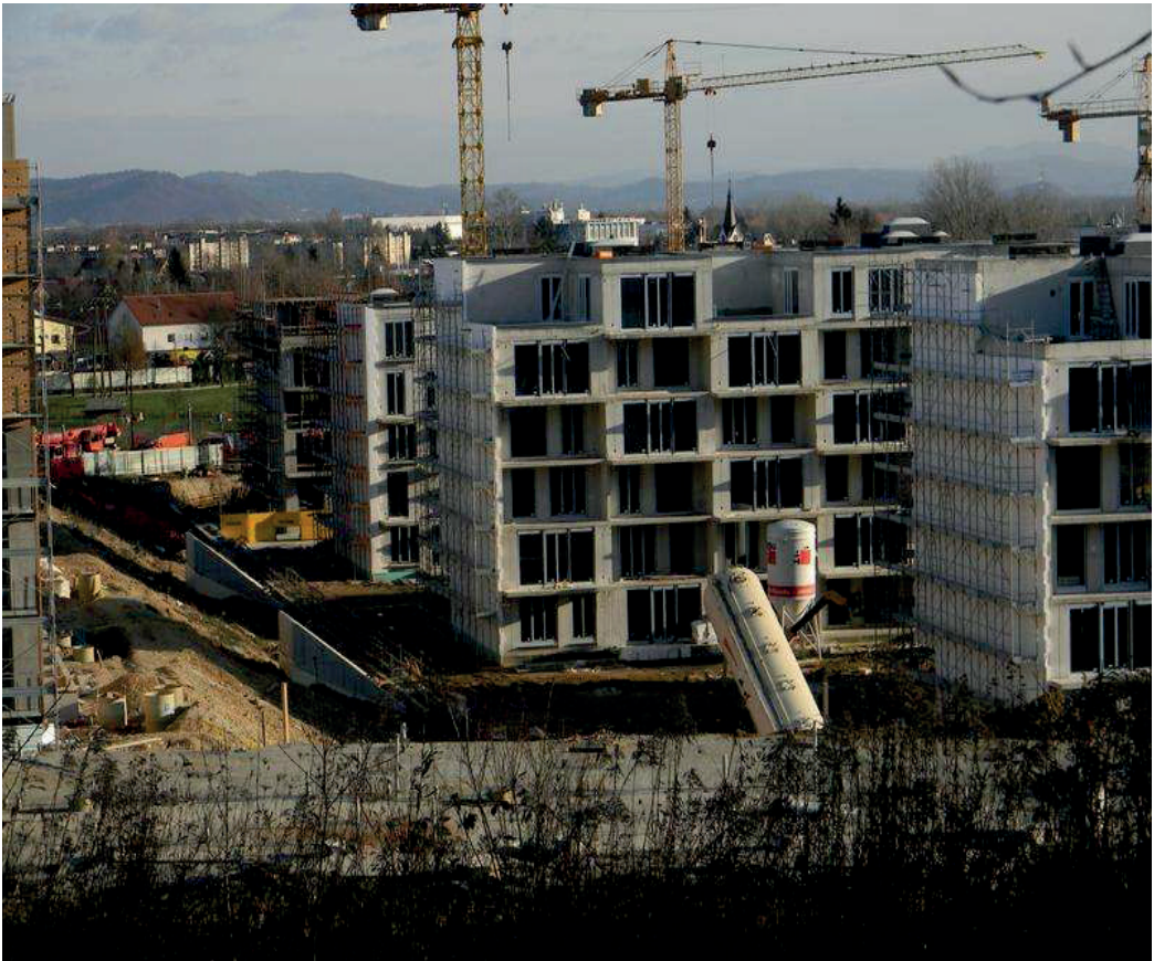
Figure 2: Example of a picture taken by a concerned citizen at the construction site and posted to the forum for other users to see the progress.
