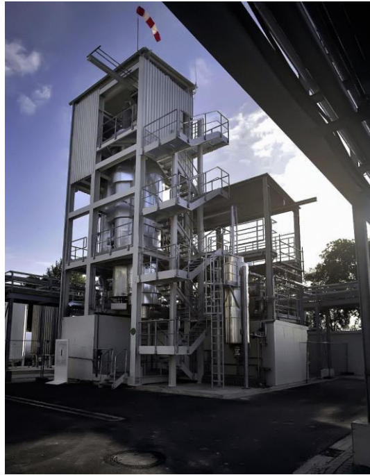
Figure 6: Methanation unit of the Audi e-gas PtG plant in Werlte. Figure taken from Audi MediaCenter [132] , Copyright © Audi AG, reproduced with permission.
