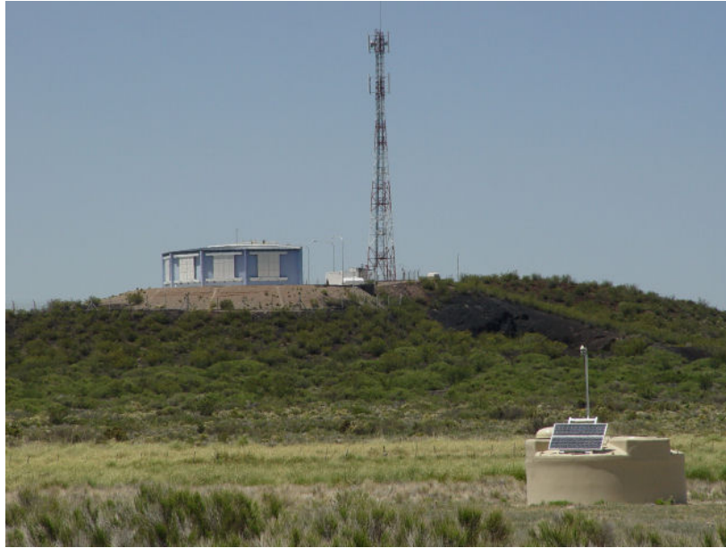
Figure 2.5 Los Leones FD building, telecommunication antenna, and an SD station.
