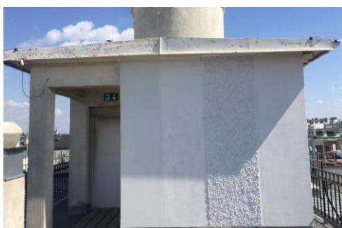
Figure 1: Tested façade, external surface after retrofit.
