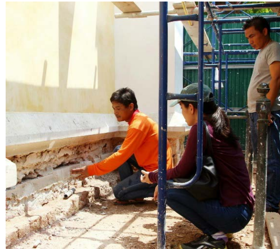
Figure 2: Last refurbishment of the temple's exterior wall in 2015.
