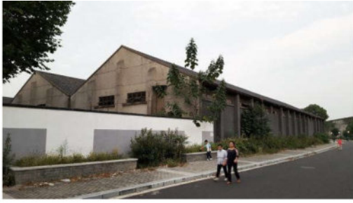
1950s_Menxi industrial area
