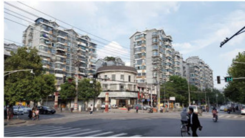
Redevelopment of highrise microdistrict in the 2000s
