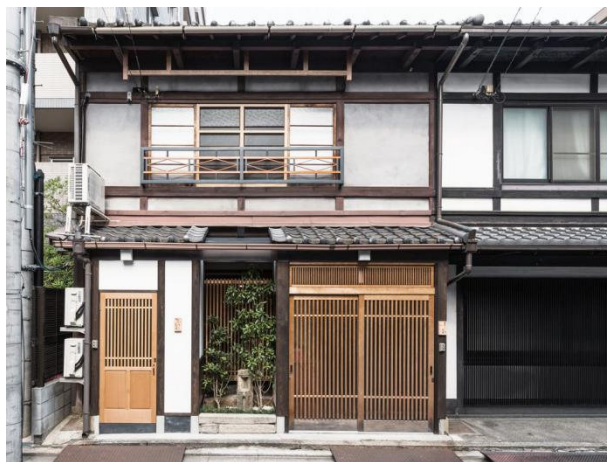
Traditional Machiya building
