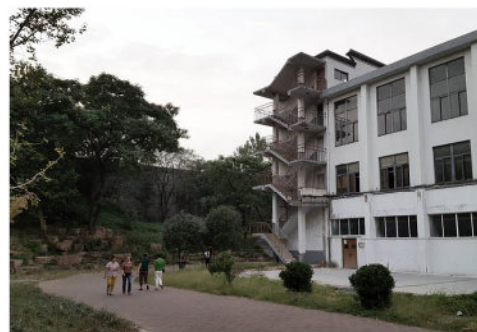
Renovation of the pedestrian along the city wall
