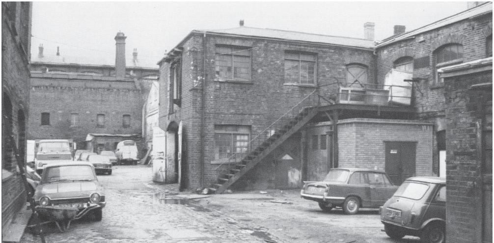
Abb. 19: Albion Yard from entrance in Balfe Street (Quelle: Angela Inglis)
